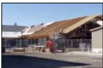
The new library wing and other classrooms in progress.
