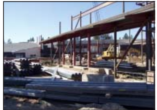
A view of the main entrance.
