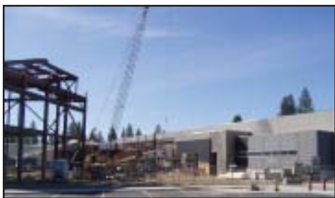
Construction view from north parking area.
