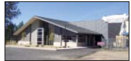
The south side addition exterior is complete.
